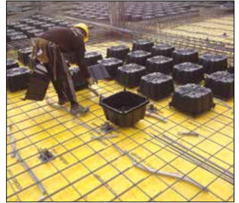
③ INSTALLATION OF NEW NAUTILUS
