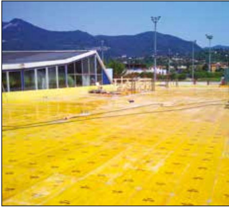
① BASE DECK PREPARATION
