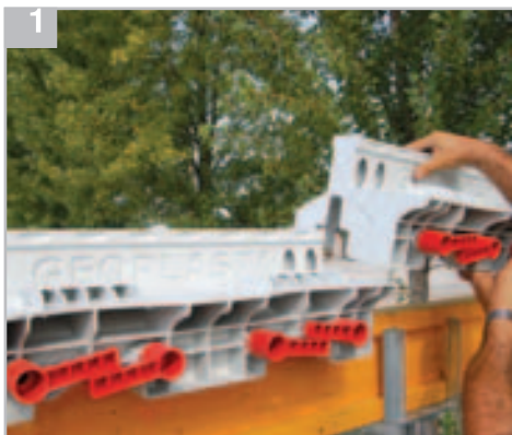
Place pre-assembled Y-beam and wedges
