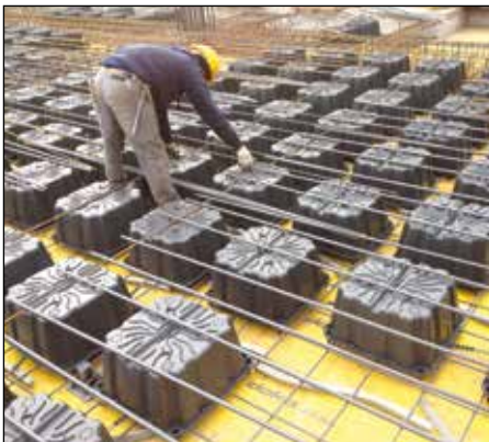
④ FINAL REINFORCE- MENT INSTALLATION
