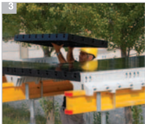
Place the GEOPANEL® 120 panel
