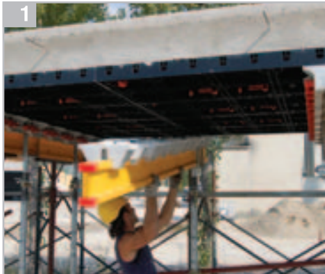
Remove the H-beams
